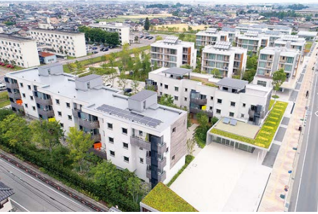
Bird's-eye view of the Passive Town project in Kurobe City, Toyama Prefecture
