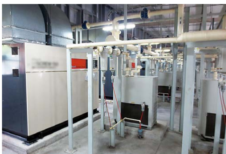
Examples of energy-saving efforts overseas Compressor in Vietnam that uses less energy by optimizing pressure (left) Checking for air leaks in Dalian, China (as well in Japan) (right)
