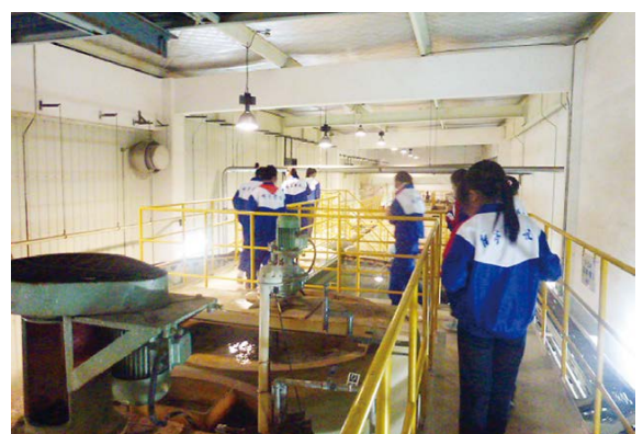
Local elementary school students tour the wastewater treatment facilities
