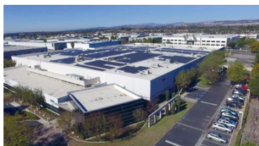
Example of installation of solar power generation equipment YKK (U.S.A.) Inc. Anaheim Plant
