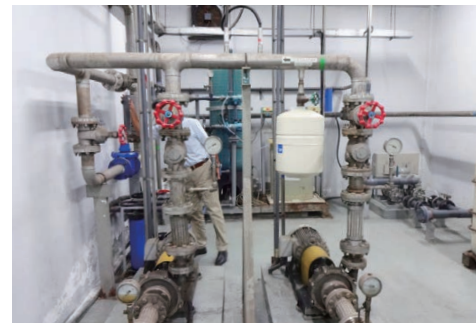
Wastewater diagnostic checking scene
