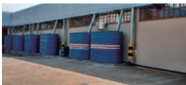
Water collection using the plant rooftop (YKK Southern Africa (Pty) Ltd.)
