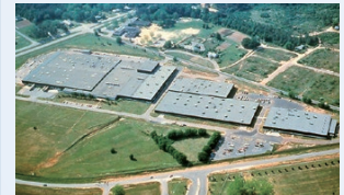
YKK (U.S.A.) Inc. Macon Plant
