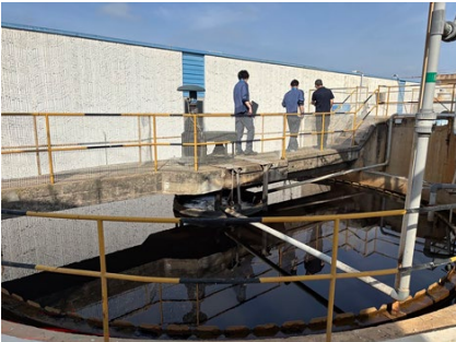
Water treatment assessment: YKK España S.A., Tortosa Factory
