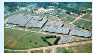
YKK (U.S.A.) Inc. Macon Plant
