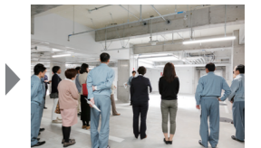
Underground parking garage. Water storage facilities are installed beneath, allowing heat from groundwater to be used in air-conditioning.
