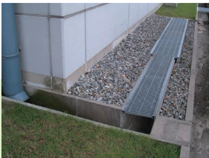
Rainwater permeable grid
