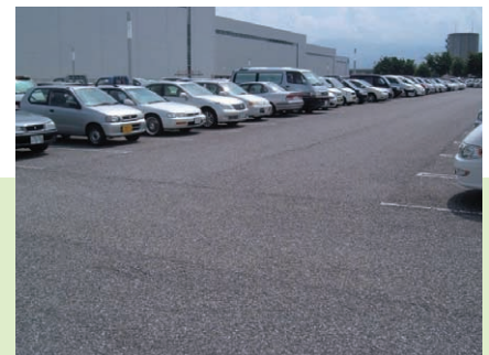
Rainwater permeable asphalt (parking lot)
