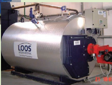
Installation of a high-efficiency boiler (YKK Hellas A.E.B.E)
