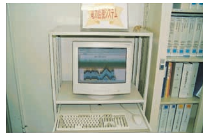
Power monitoring system
