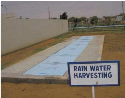
Rainwater harvesting equipment at YKK India
