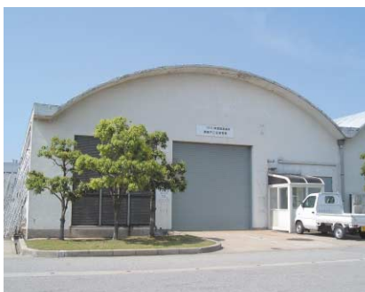
Storage warehouse for equipment that contains small amounts of PCBs
