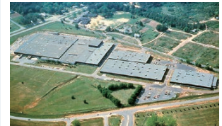
YKK (U.S.A.) Inc. Macon Plant
