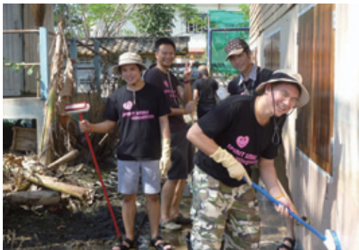
Cleaning submerged facilities
