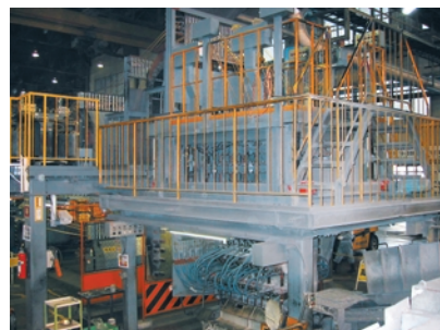
New molding line
