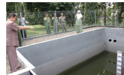
Depok City mayor observing a rainwater storage and infiltration facility
