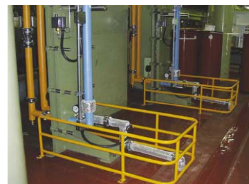
New indoor heat exchanger
