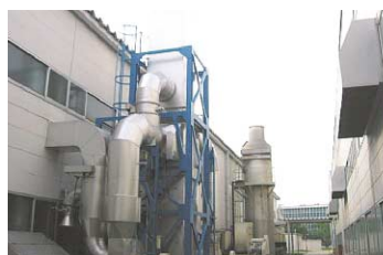
Combustion furnace for paint gas emissions at the Fastening Products Group plant
