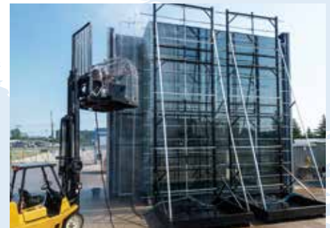
Unit curtain wall performance verification by Erie AP
