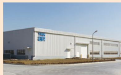
The new door and window manufacturing plant
