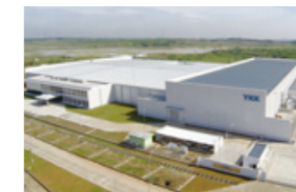
PT YKK ZIPCO INDONESIA's new copper alloy wire plant
