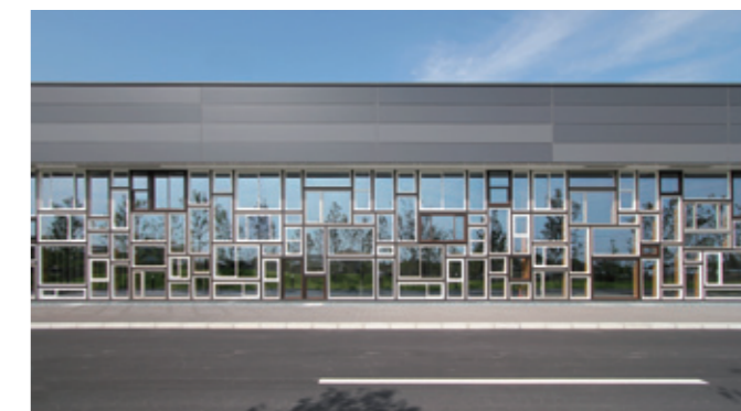
The plant's office building boasts approximately 300 sets of APW 330 heat insulation windows (Photo by Takenaka Corporation)
