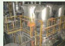
Burner's refractory replacement
