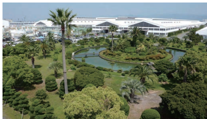
YKK AP Inc. Kyushu Plant
