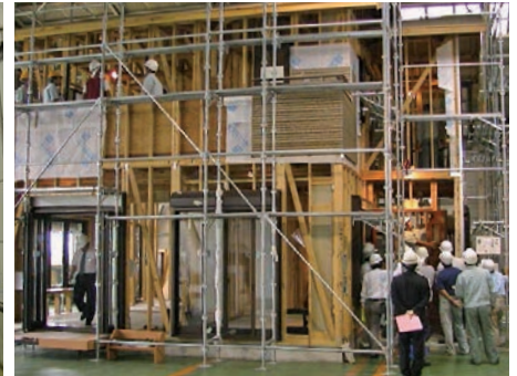
Implementation of training for builders to prevent accidents
