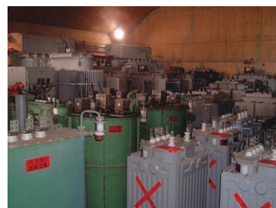
Dedicated storage warehouse for equipment that contains small amounts of PCBs
