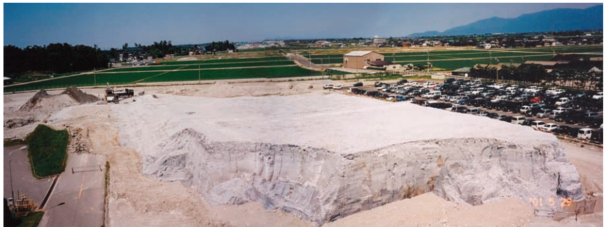
May 2001: Digging out carbide sludge (mid-process)
