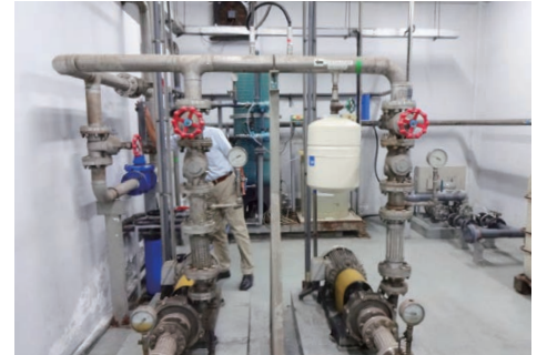
Wastewater diagnostic checking scene
