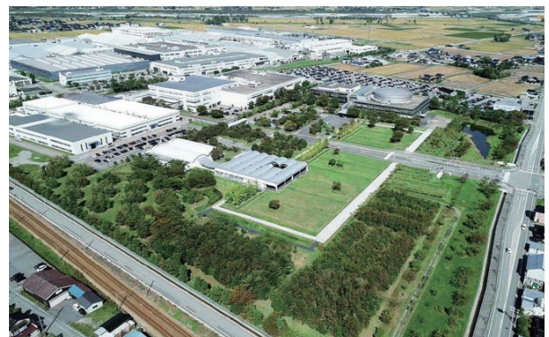
YKK Center Park (Kurobe City, Toyama Prefecture)
