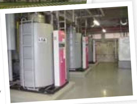
High efficiency once-through boilers
