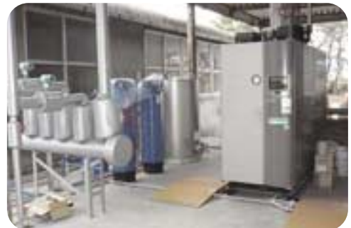
Boiler fuel conversion (heavy oil → natural gas)
